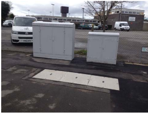
Construct Range4 New NTL Cabinet
